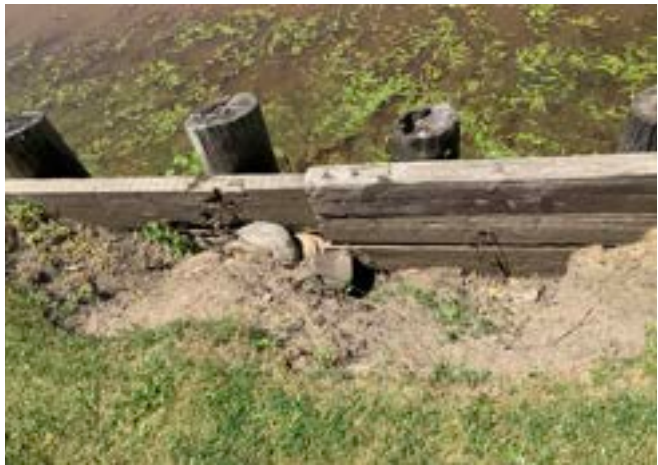
Figure 5.7: Failing Timber Wall (1)
