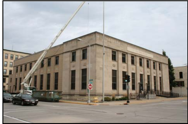
U.S. Post Office (1937) at 19 W. 1 st Street.
