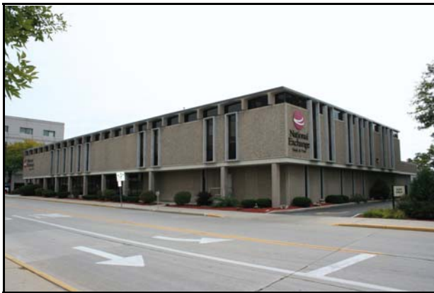
130 S. Main Street: National Exchange Bank & Trust
