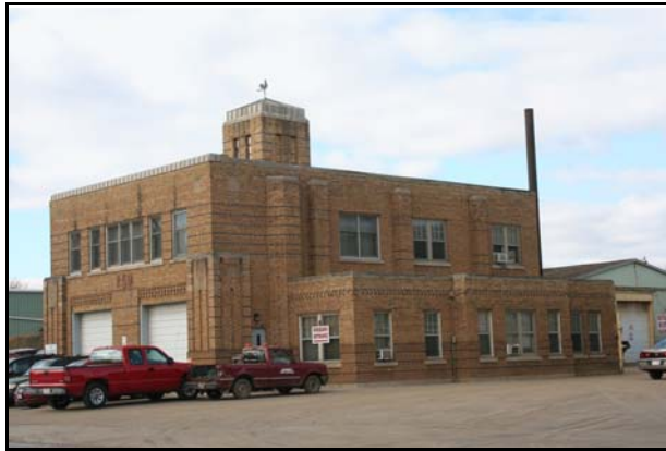
251 W. Arndt Street: Fond du Lac Fire Department Hose Company #3 (November 2010)
