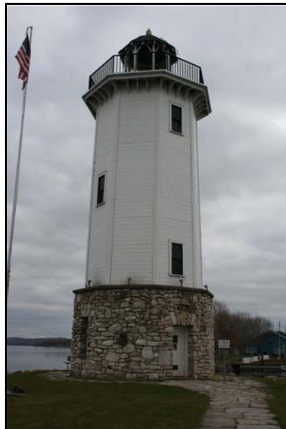
Lakeside Park Lighthouse
