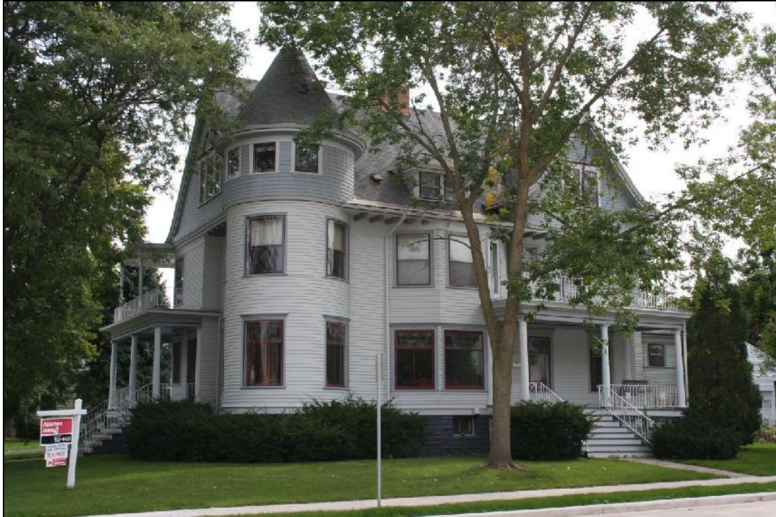
S. Park Avenue elevation (2010 photo)
