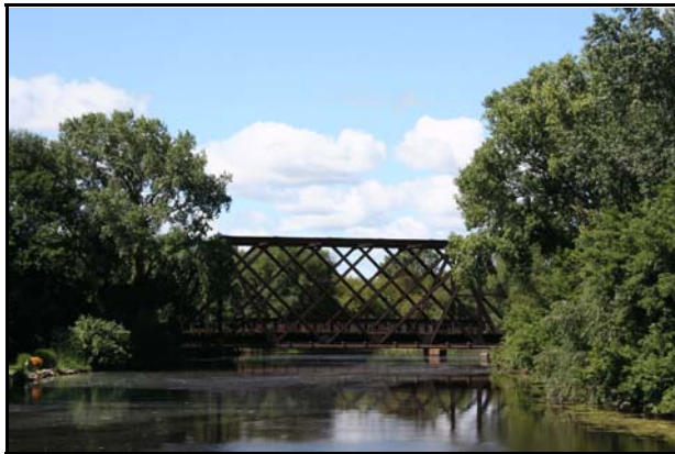
South of Scott Street: Chicago & North Western Railroad Bridge
