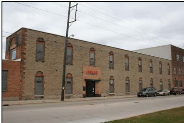
2-26 S. Brooke Street: LaBelle Wagon Works/Gurney Refrigerator Company
