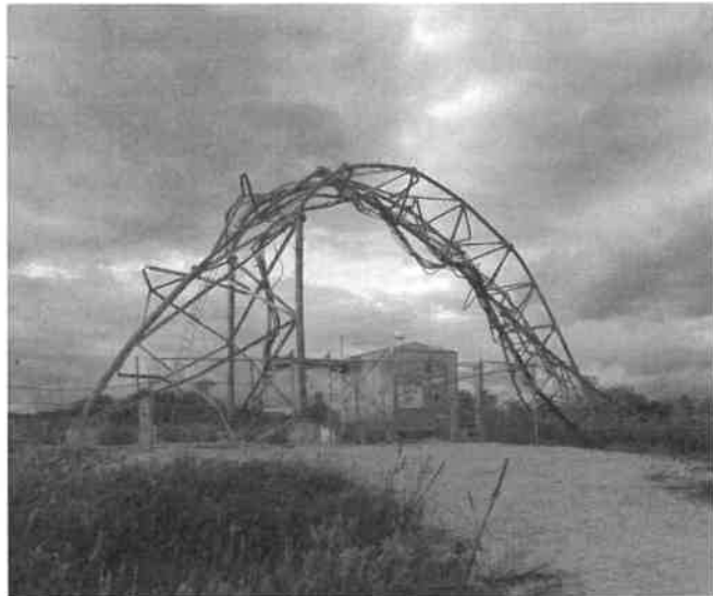
Tornado damage west of Brownsville, Fond du Lac County, August 28, 2018. Source: National Weather Service, Milwaukee/Sullivan, WI Weather Forecast
