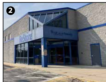
13 W Scott St Minor Improvements Needed
