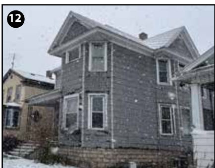
12 27 E Johnson St Major Improvements Needed
