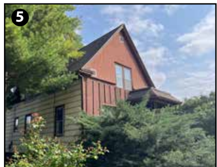
321 N Macy St Major Improvements Needed
