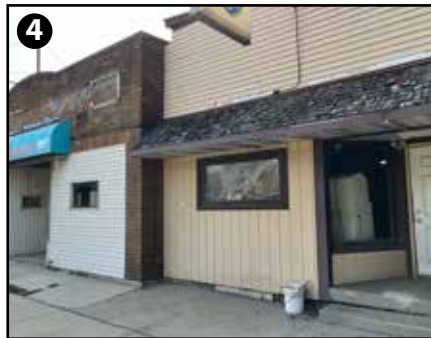
234 N Main St Minor Improvements Needed
