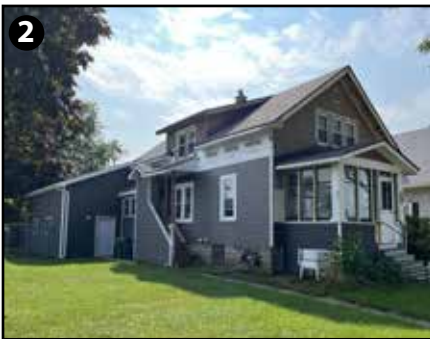
30 W Scott St Minor Improvements Needed
