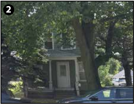
26 W McWilliams St Minor Improvements Needed
