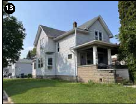
13 398 N Main St Minor Improvements Needed
