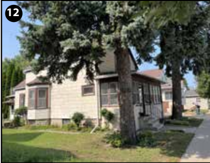
12 402 N Main St Minor Improvements Needed
