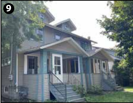
9 30 W Bank St Minor Improvements Needed
