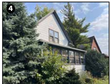
323 N Macy St Major Improvements Needed
