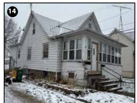
14 190 Marquette St Minor Improvements Needed
