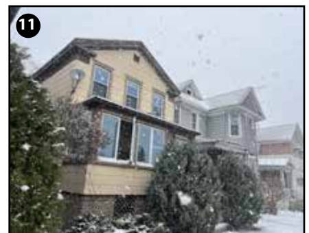
11 25 E Johnson St Major Improvements Needed
