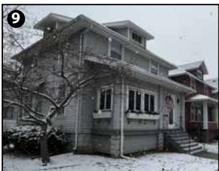
9 42 E Follett St Minor Improvements Needed
