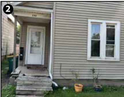
246 N Main St Minor Improvements Needed
