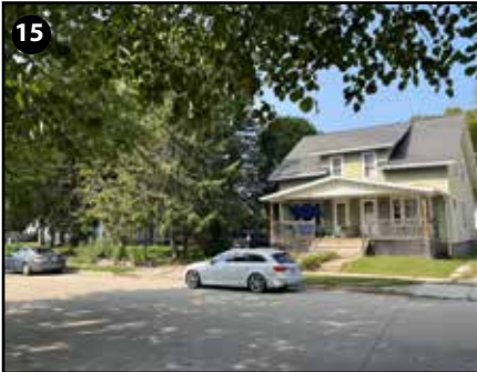
15 35 W McWilliams St Minor Improvements Needed
