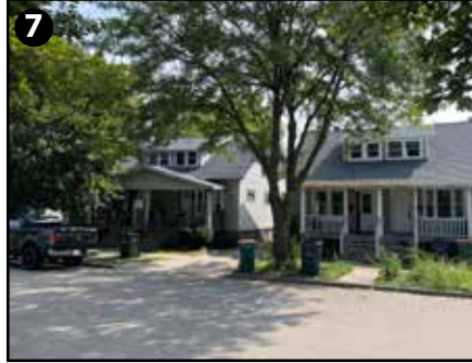
7 38 W Bank St Minor Improvements Needed
