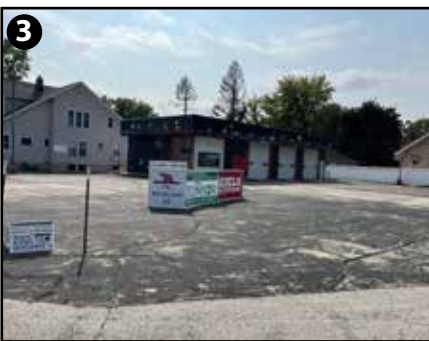
446 N Main St Major Improvements Needed
