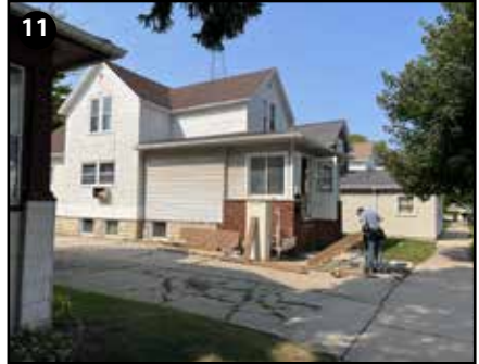
11 408 N Main St Minor Improvements Needed
