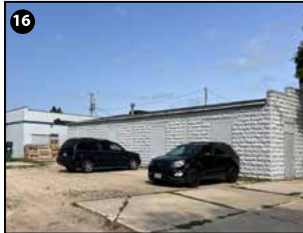
16 17 W McWilliams St Major Improvements Needed
