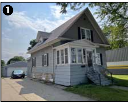
34 W Scott St Minor Improvements Needed
