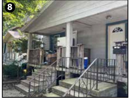
8 34 W Bank St Minor Improvements Needed
