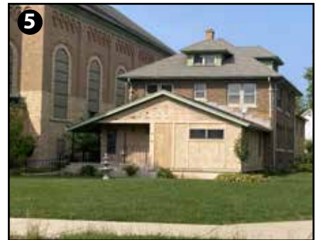
37 E Follett St Minor Improvements Needed
