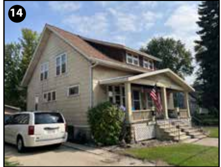
14 377 N Macy St Minor Improvements Needed
