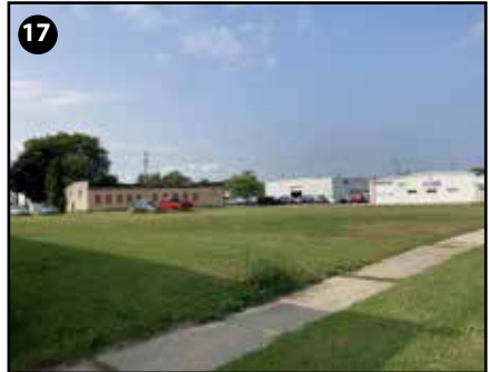
17 365 N Main St Major Improvements Needed
