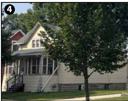
37 W Bank St Minor Improvements Needed
