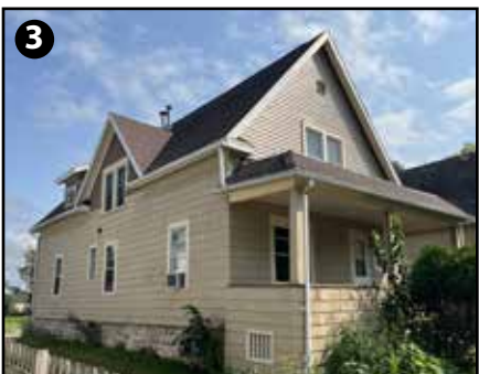
333 N Macy St Minor Improvements Needed
