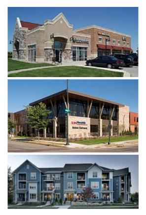
Examples of various techniques in use to break down the apparent mass of a large building, including canopies, recessed decks, recessed top story, and variations in materials and wall plane.
