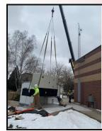
FDLFR Station 1 replaced its emergency generator. The new generator will have greater capacity and provide better reliability than the original unit which had reached the end of its service life.
